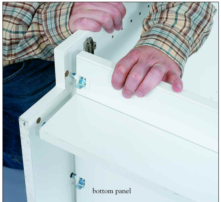
7 Attach the left side by aligning the pre-drilled holes with the connection fittings in the back, bottom and top panels.
