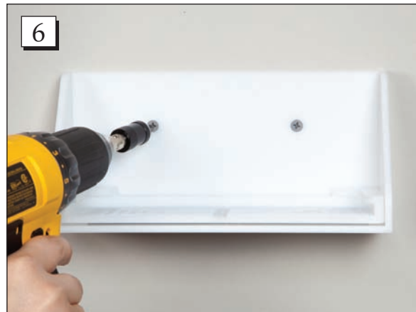
Step 6. Once level, tighten screw into the remaining hole.
