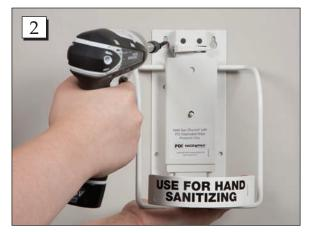
**Step 2.** Place a screw in the first mounting hole and tighten the screw with a screwdriver. Repeat with the remaining three mounting holes.
