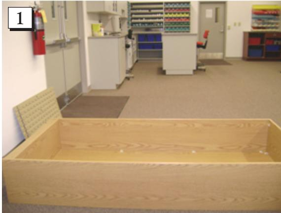
**Step 1.** Start by laying the cabinet down on the floor.
