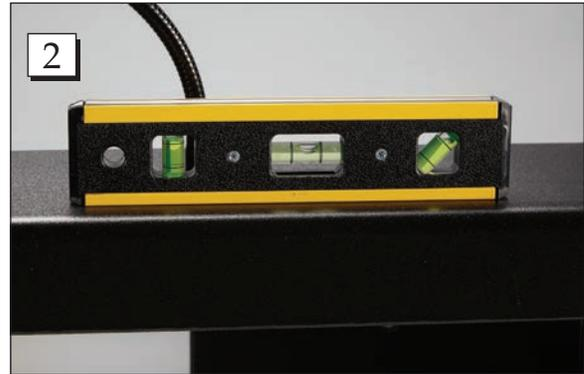
**Step 2.** Once your box is attached using one of the four keyholes, level the box and install hardware in the three remaining keyholes.
