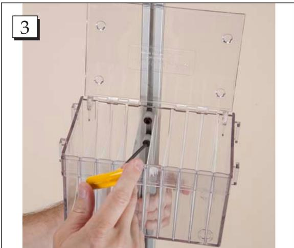
**Step 3.** Tighten the screws on all of the T-Nuts.
